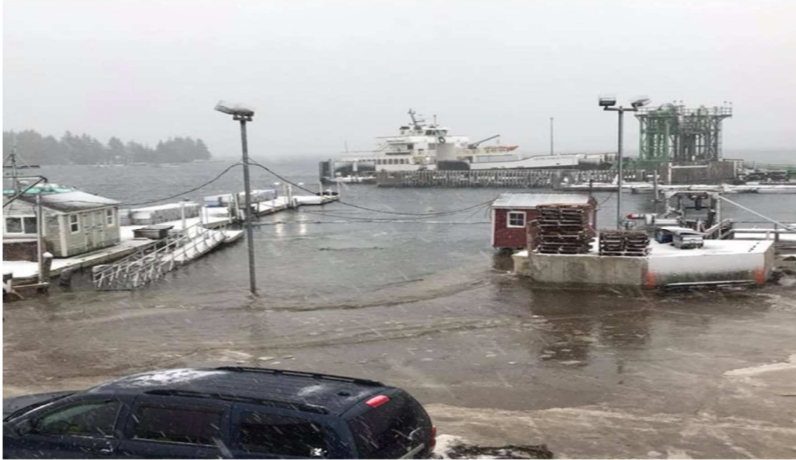
January 4, 2018 Winter Storm Grayson. Vinalhaven's Carvers Harbor southeast exposure. Pictured here is a lobster buying station with no pedestrian access due to storm tides. In the background is a Maine State Ferry Service boat in its pen. Photo: Andrew Dorr
